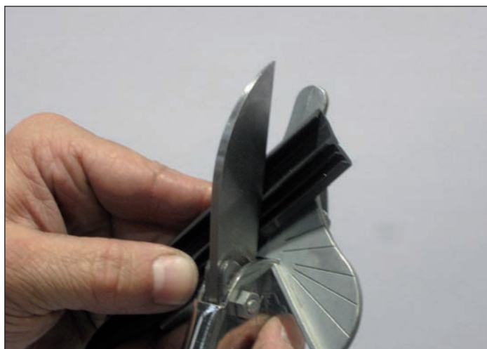
Fig. 285 Cutting the rebate glazing weatherstrip
