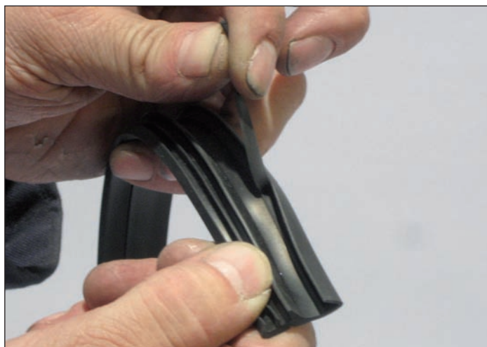
Fig. 284 Removing the tear-off lips before installation
