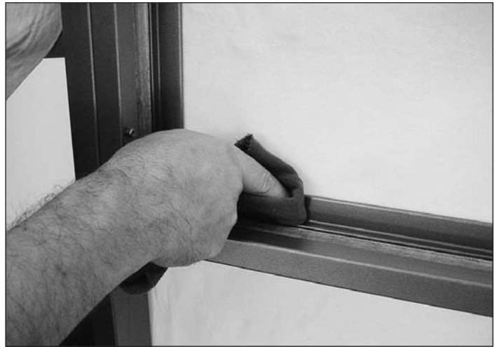
Fig. 274 Cleaning the profile rebate
