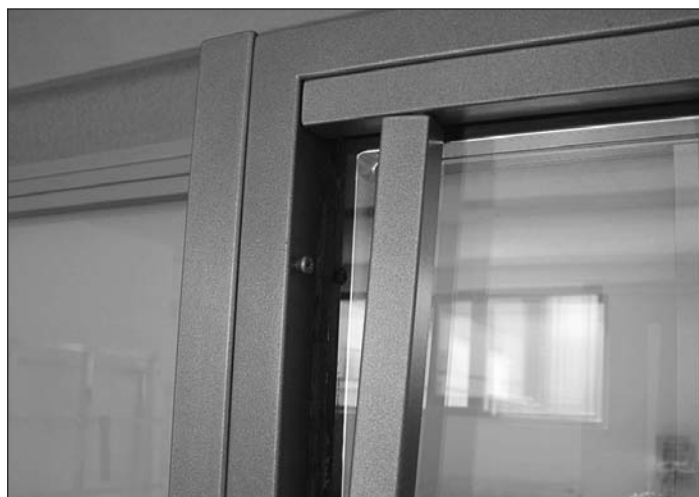
Fig. 279 Installing the glazing beads
