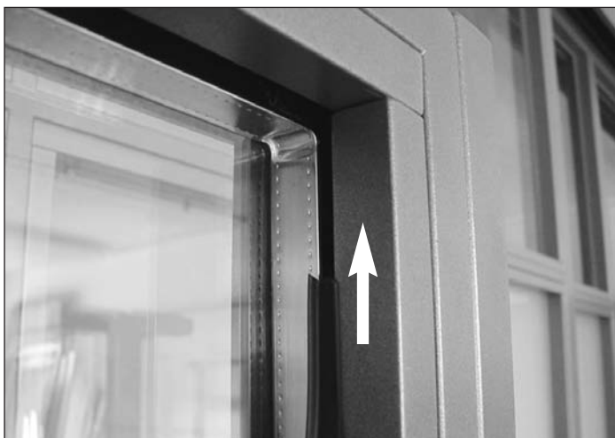
Fig. 281 Pressing in the glazing weatherstrip
