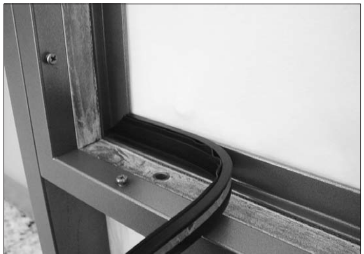
Fig. 276 Installing the external glazing weatherstrip
