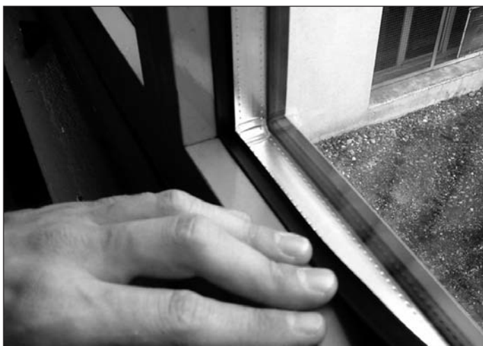
Fig. 282 Installing the inner glazing weatherstrip
