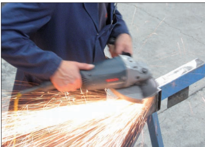
Fig. 130 Machine the welded corner from inside to outside
