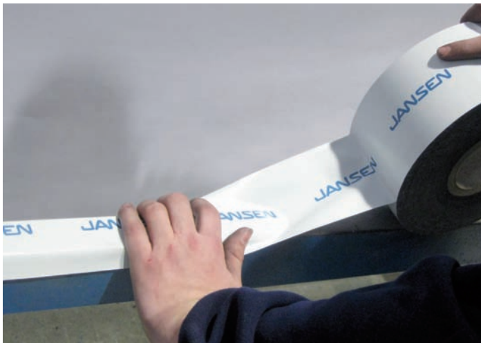
Fig. 204 Mask the trestles with protective foil
