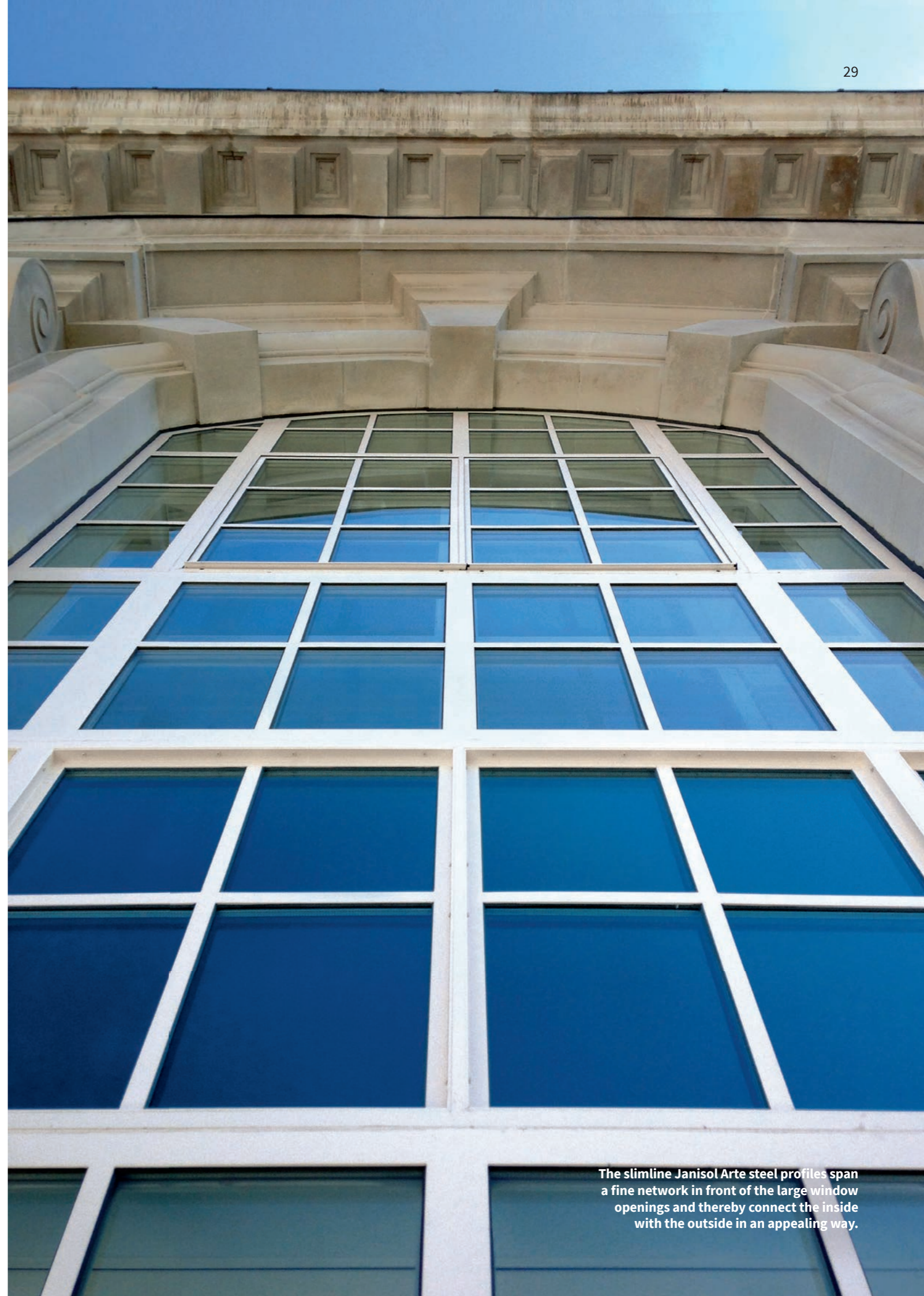
The architects opted to update the large window areas in keeping with the old style using steel profile systems.
