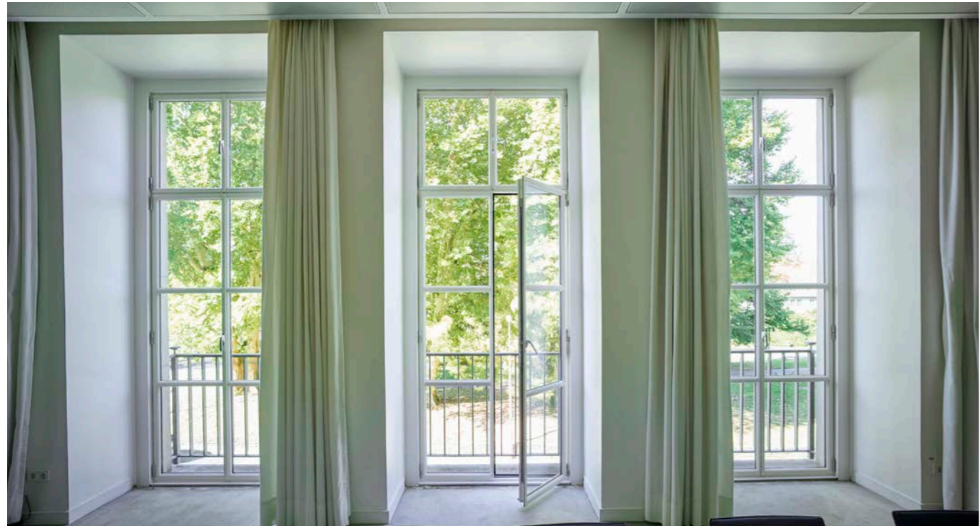
The three window doors in the meeting room of the council groups (Europazimmer) were reconstructed using the Janisol Arte 2.0 steel profile system, following the example of the original fenestration of the 1950s.
